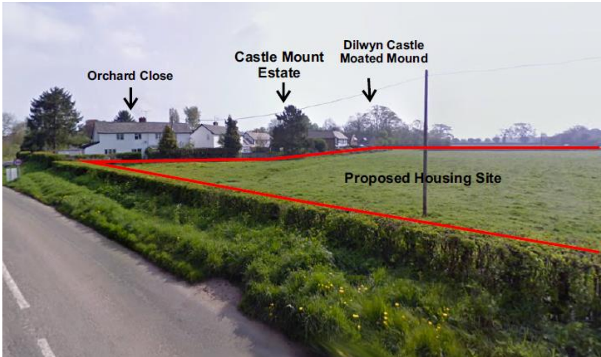
Figure 5: Closer view across proposed housing site towards Dilwyn Castle Moated Mound from the south-west.
